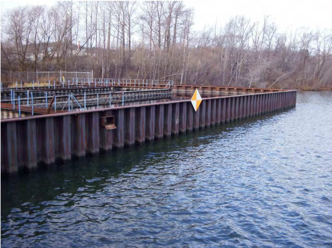
Photo 2 – Overall View of East Wall
