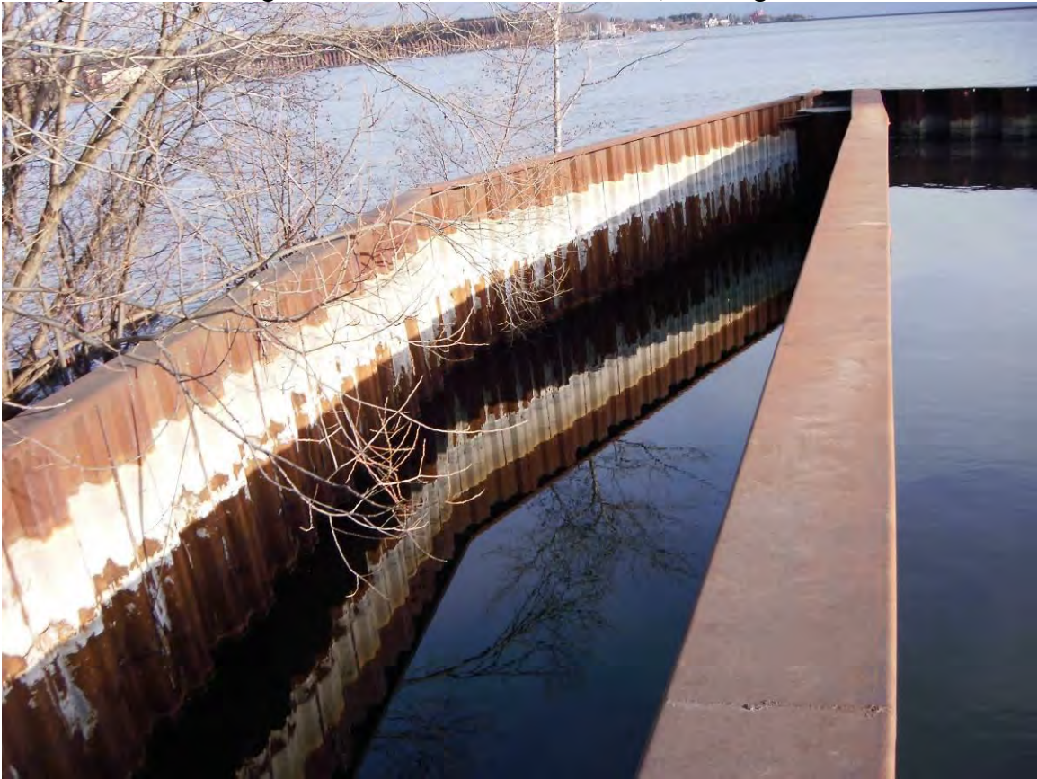
Photo 3 – Recently Constructed North Sheet Pile Wall
