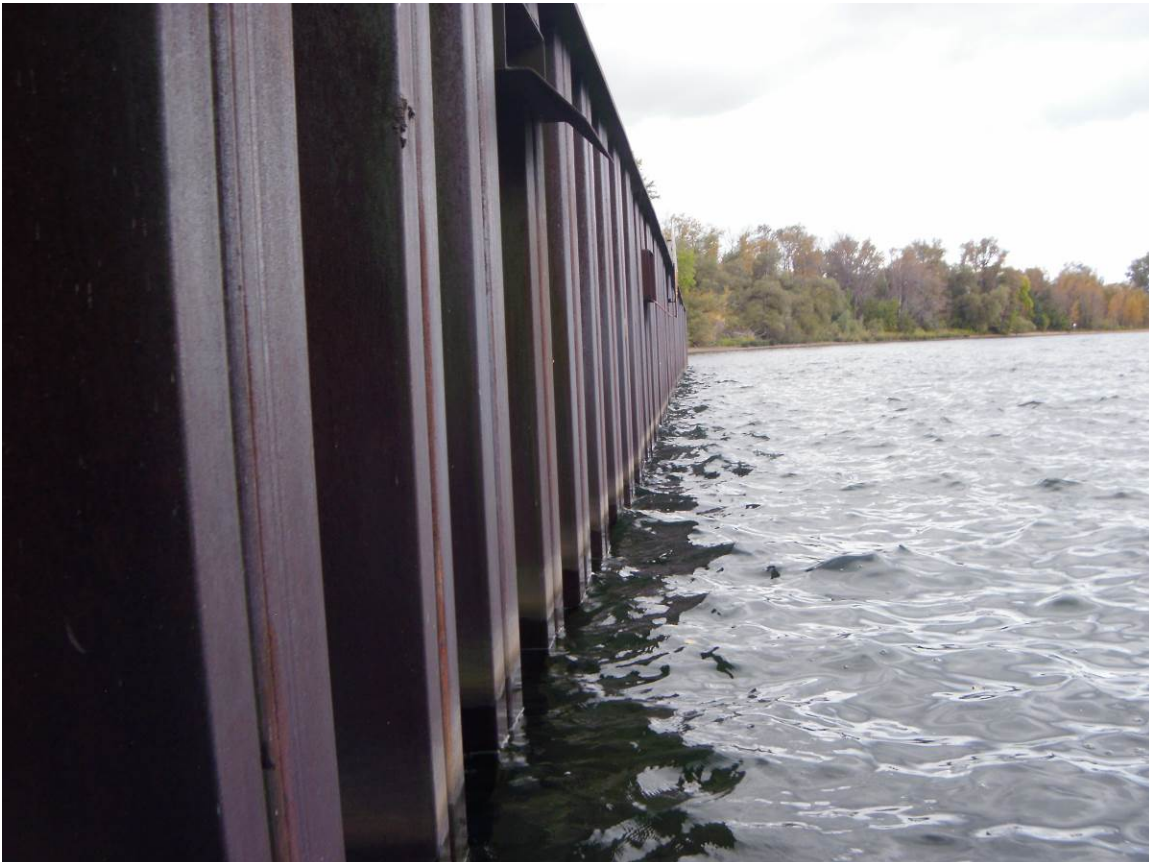
Photo 2 – Overall View of East Wall
