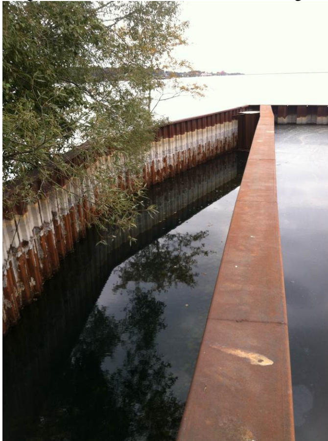
Photo 3 – Recently Constructed North Sheet Pile Wall
