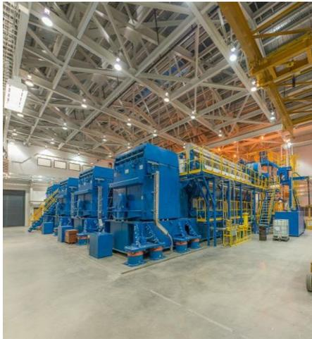
The new Marquette Energy Center will consist of three 17 megawatt Wartsila reciprocating internal combustion engines.
