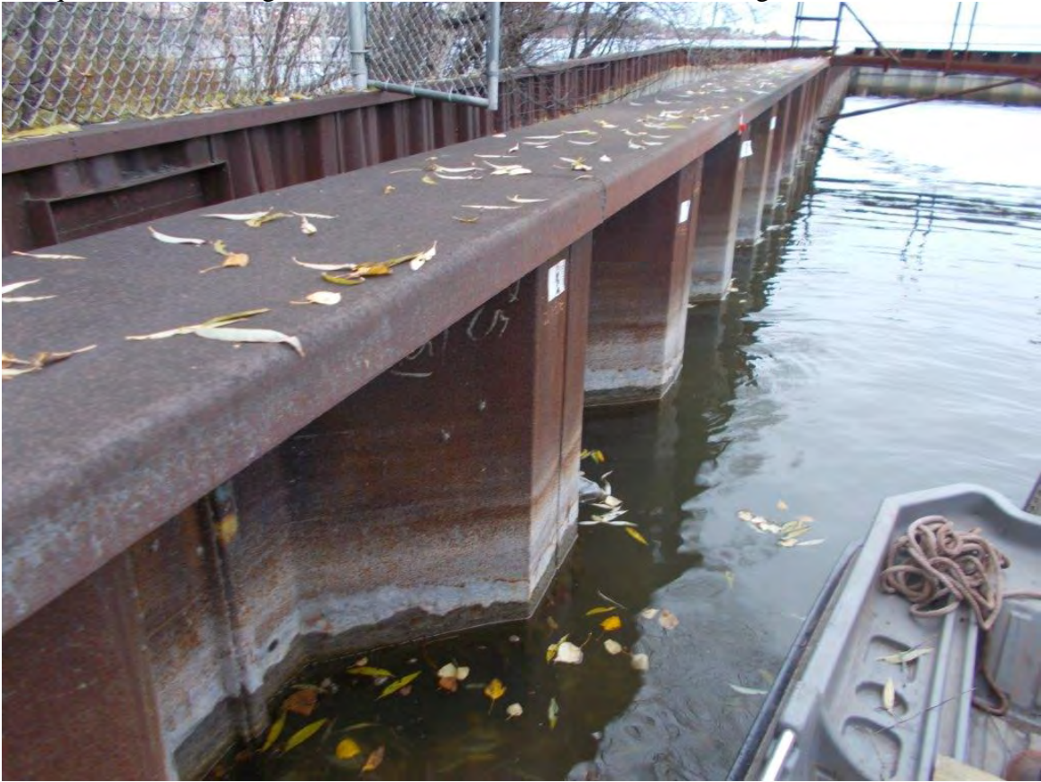
Photo 3 – Recently Constructed North Sheet Pile Wall
