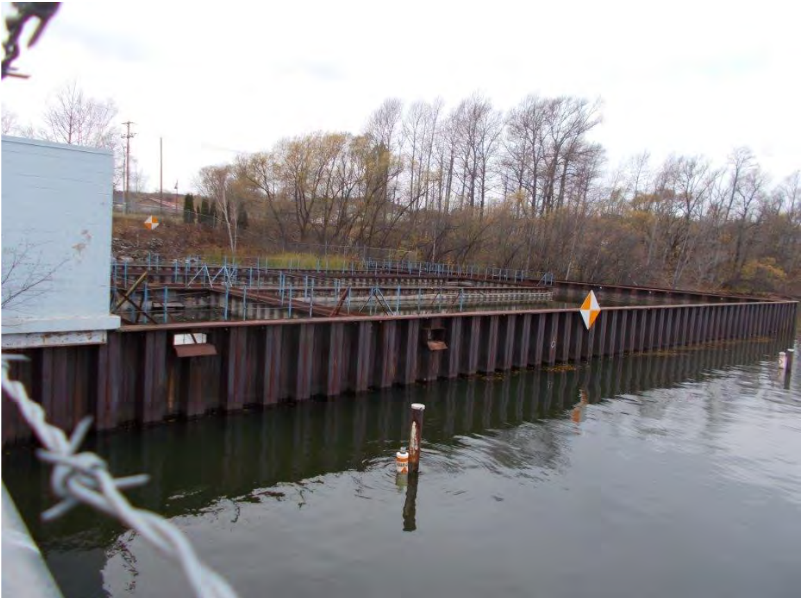
Photo 2 – Overall View of East Wall
