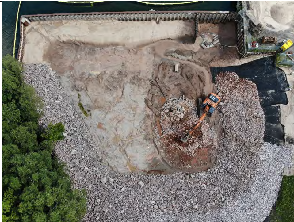
Photo No. 28 – September 4, 2020 – Overall Final Subgrade
