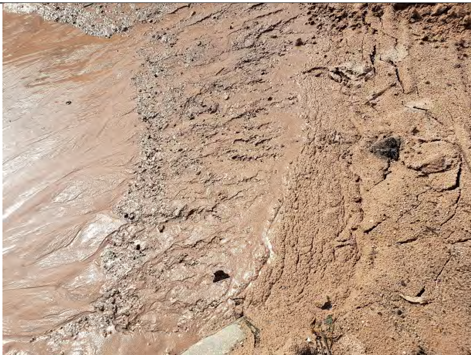
Photo No. 24 – September 1, 2020 – Final Subgrade Sample #13
