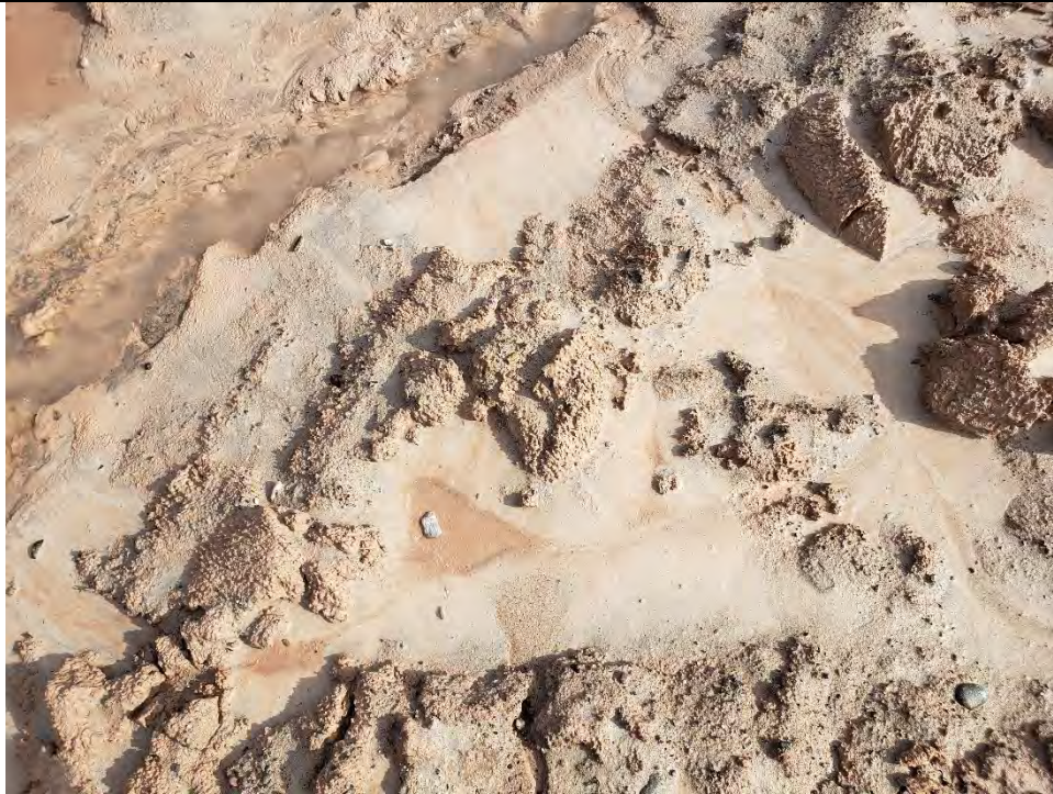
Photo No. 21 – September 1, 2020 – Final Subgrade Sample #10
