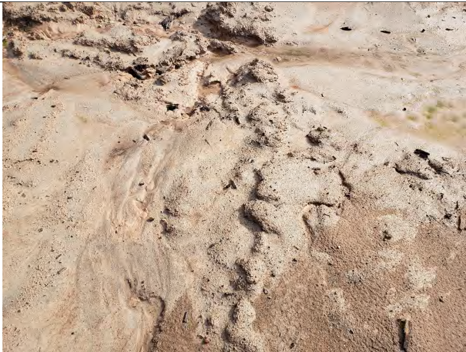
Photo No. 20 – September 1, 2020 – Final Subgrade Sample #9
