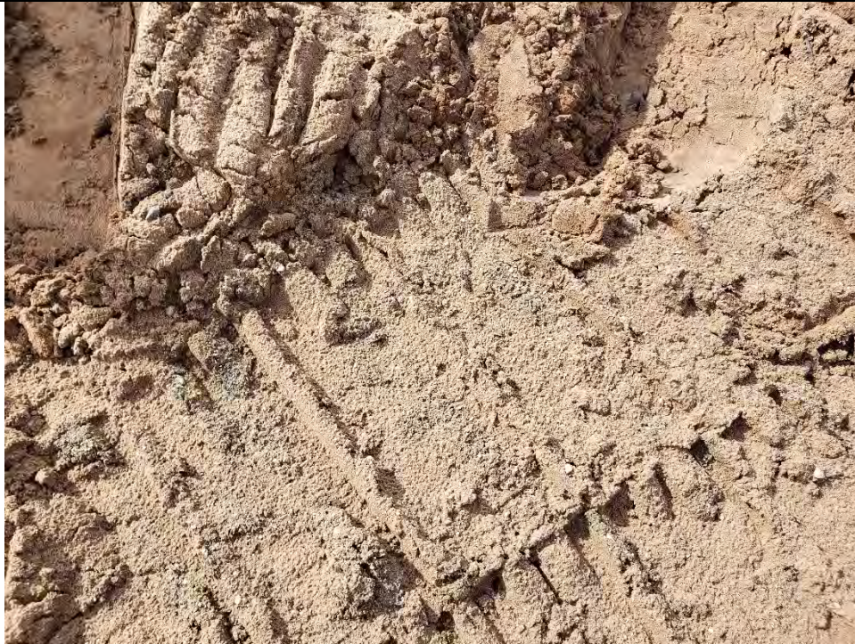
Photo No. 25 – September 1, 2020 – Final Subgrade Sample #14
