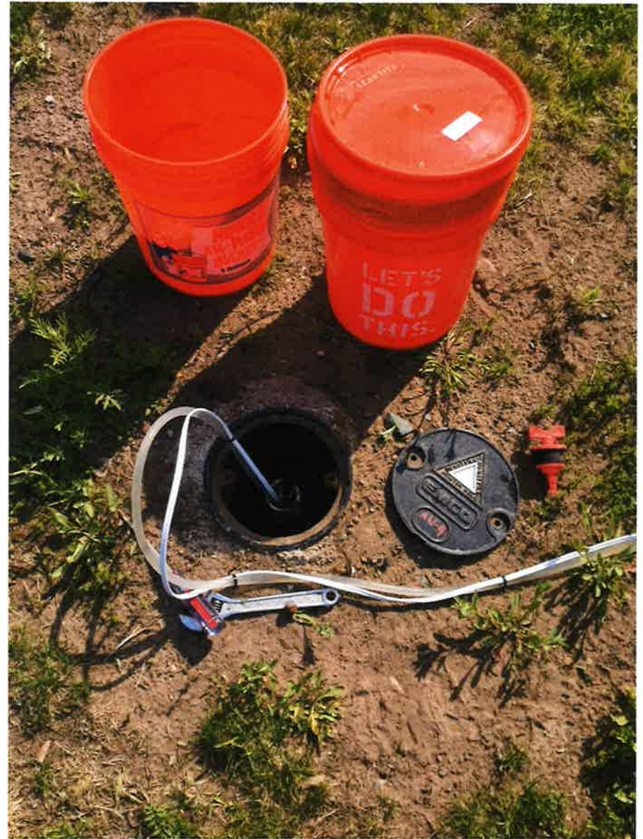
Well development (MW-4)
