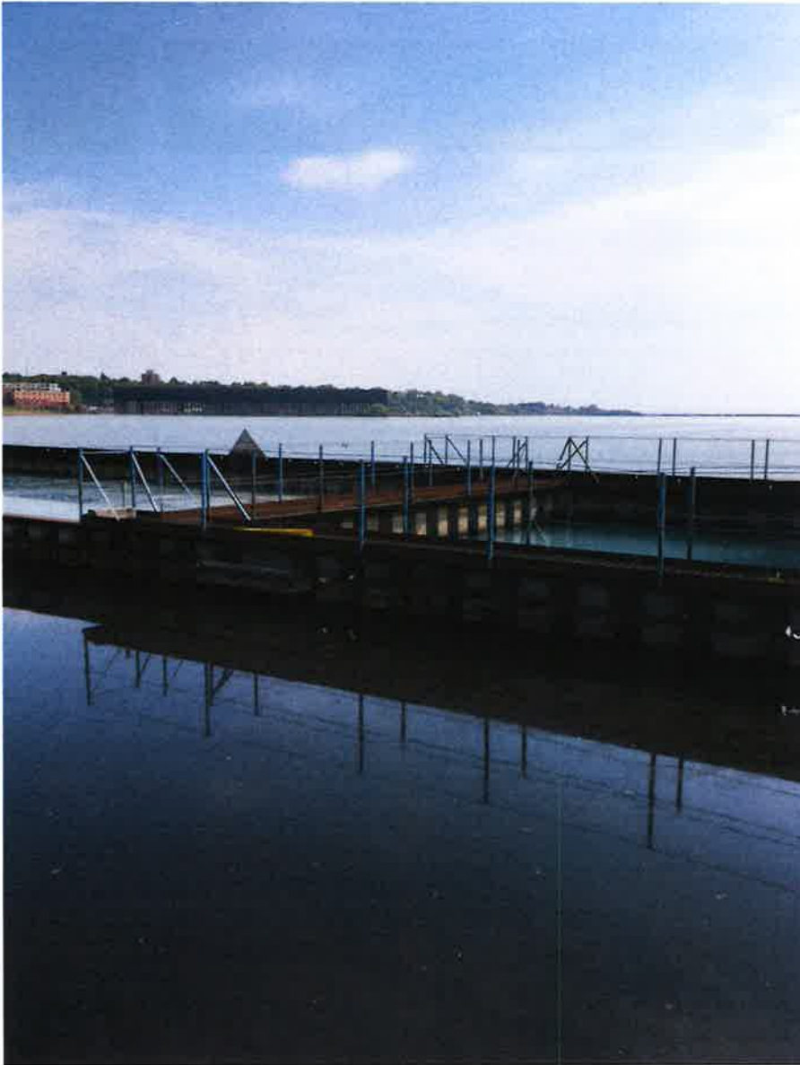
Retention ponds, facing NNW.
