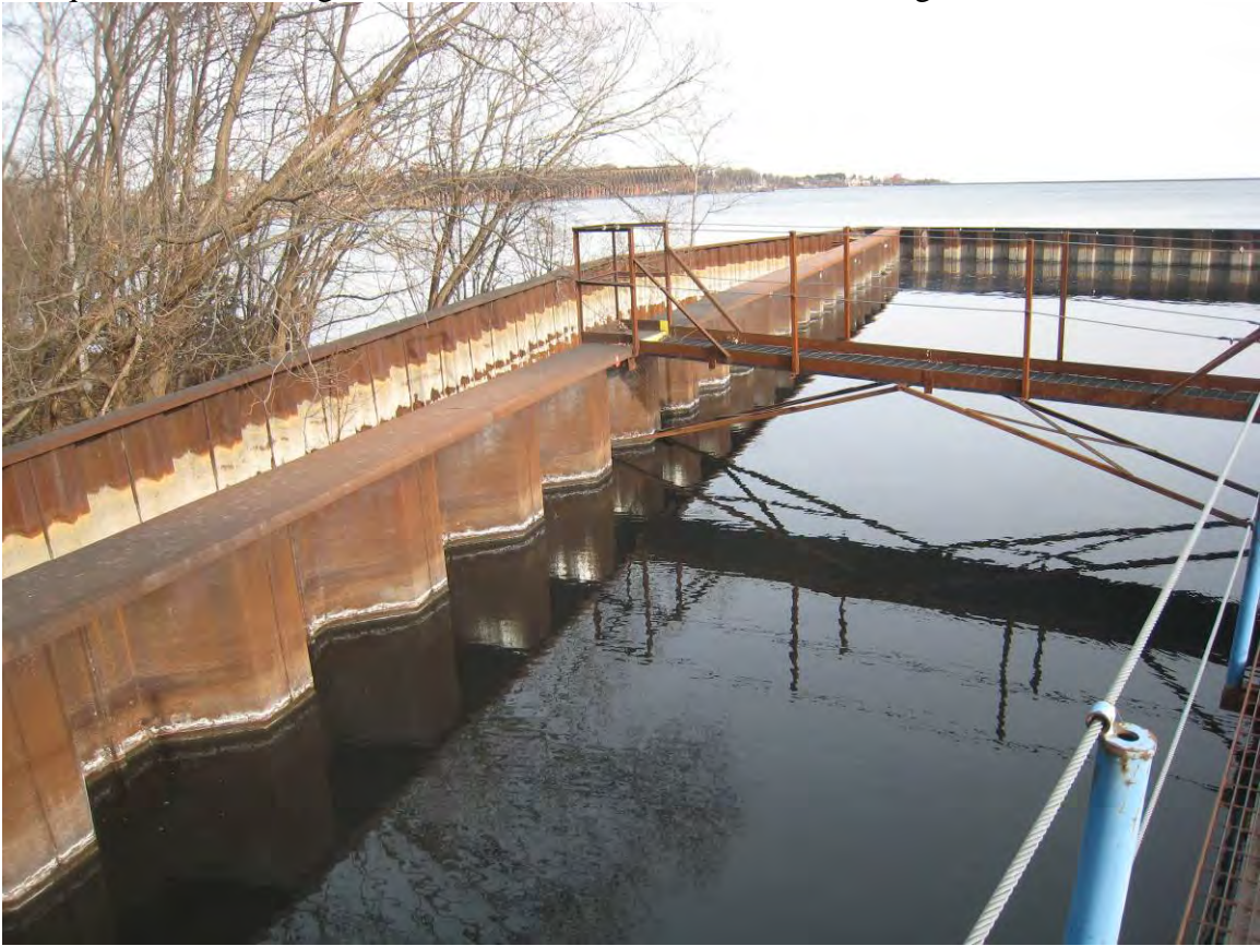
Photo 3 – Recently Constructed North Sheet Pile Wall
