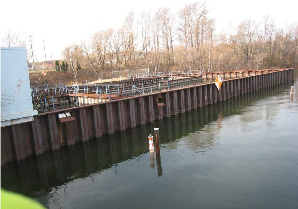
Photo 2 – Overall View of East Wall
