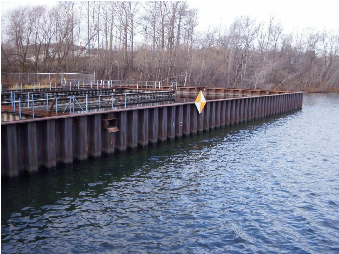
Photo 2 – Overall View of East Wall
