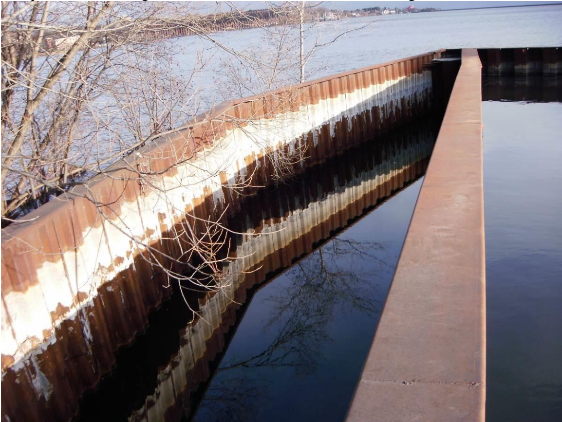
Photo 3 – Recently Constructed North Sheet Pile Wall
